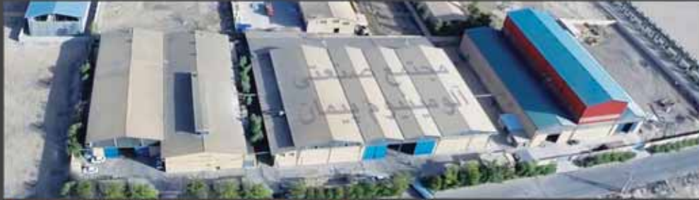
Peyman Aluminium Industrial Complex
