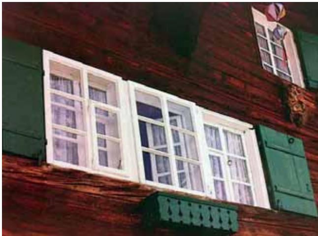
BOX-TYPE WINDOWS IN MÜRREN, SWITZERLAND
